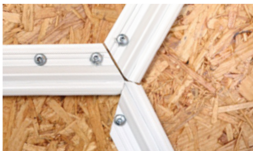
Image B11 - example of connection of three profiles - shell
